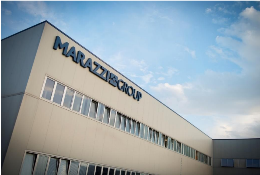
Marazzi Group – Plant of Fiorano Modenese
